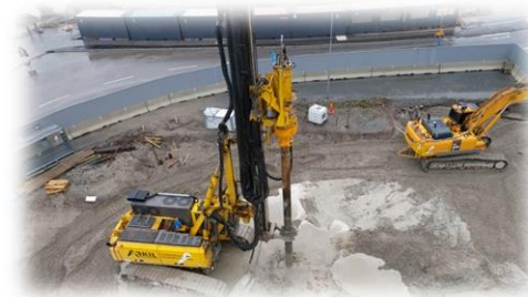
Soil mixing / cement stabilisering
