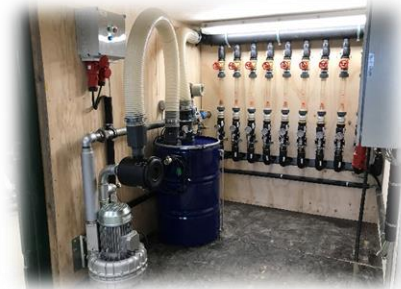
Air sparging / ventilation
